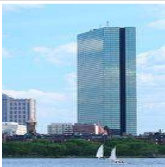
Figure 5: Image of the John Hancock Tower in Boston, MA, USA
